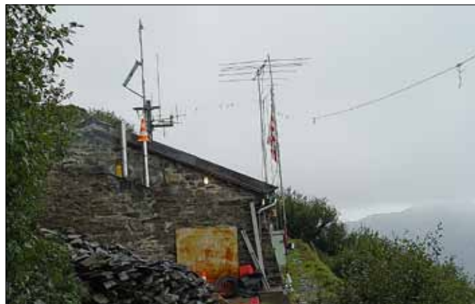
Antennen - HF: Kelemen / 6m: Tonna / 2m - 23cm: Vertical
