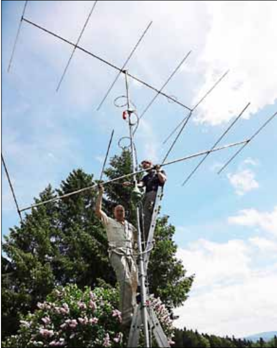
Antennenbau: Pierre-André HB9FMN, oben Stan HB9FMT
