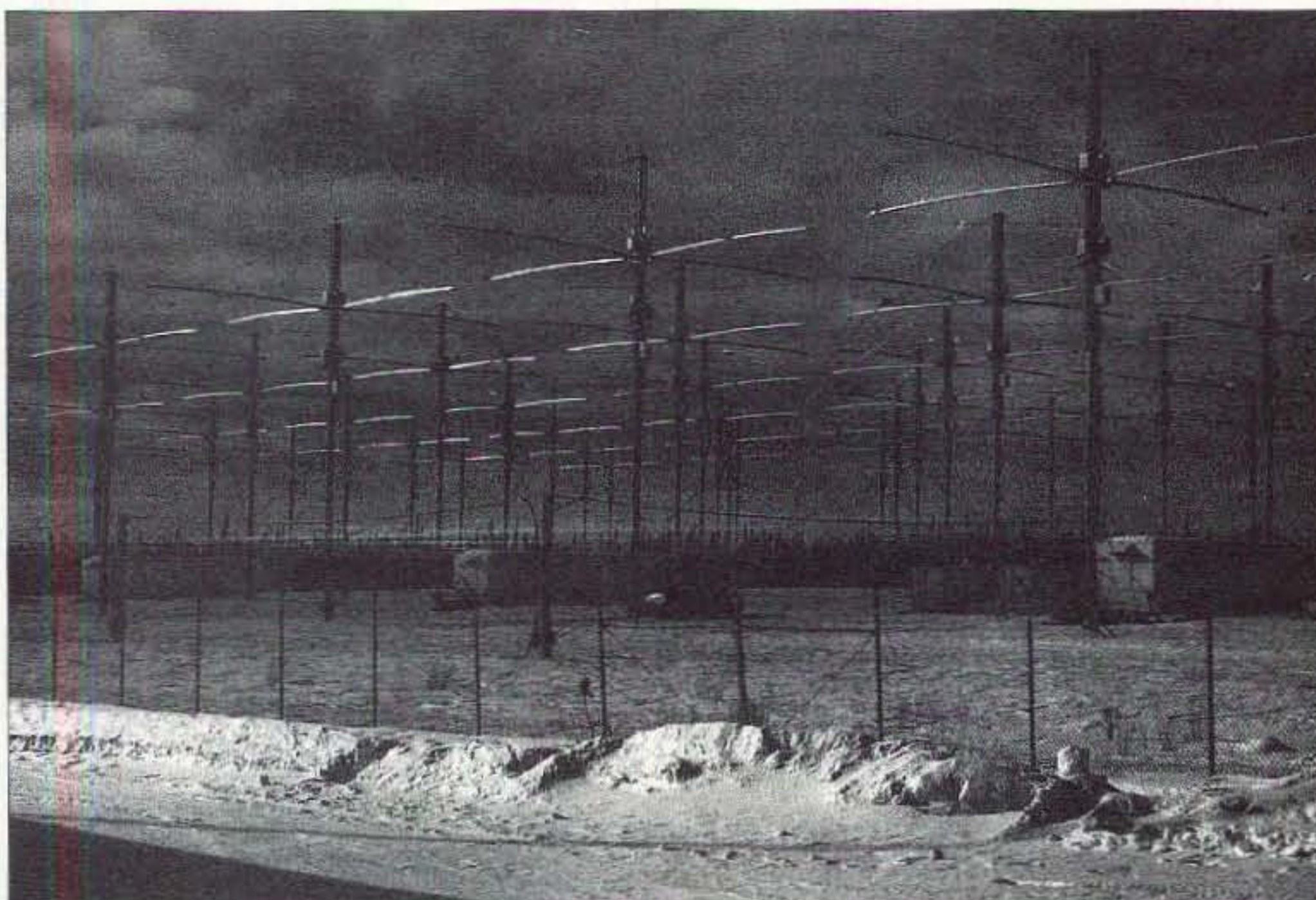
Photo A. Classic view of the HAARP antenna field. Transmitters are housed in the large white vans.
