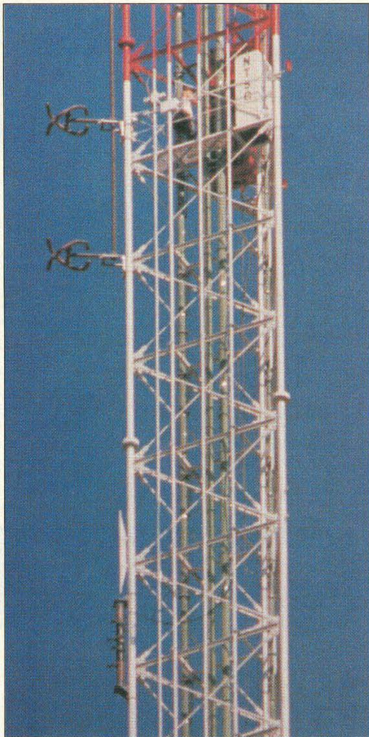
Photo A. The NTSC ATV repeater is situated at the 1270-foot level of a commercial TV tower near the Dallas-Ft. Worth area. Photo taken by Robert Skegg VE7AII/W5 through a high-power lens.
