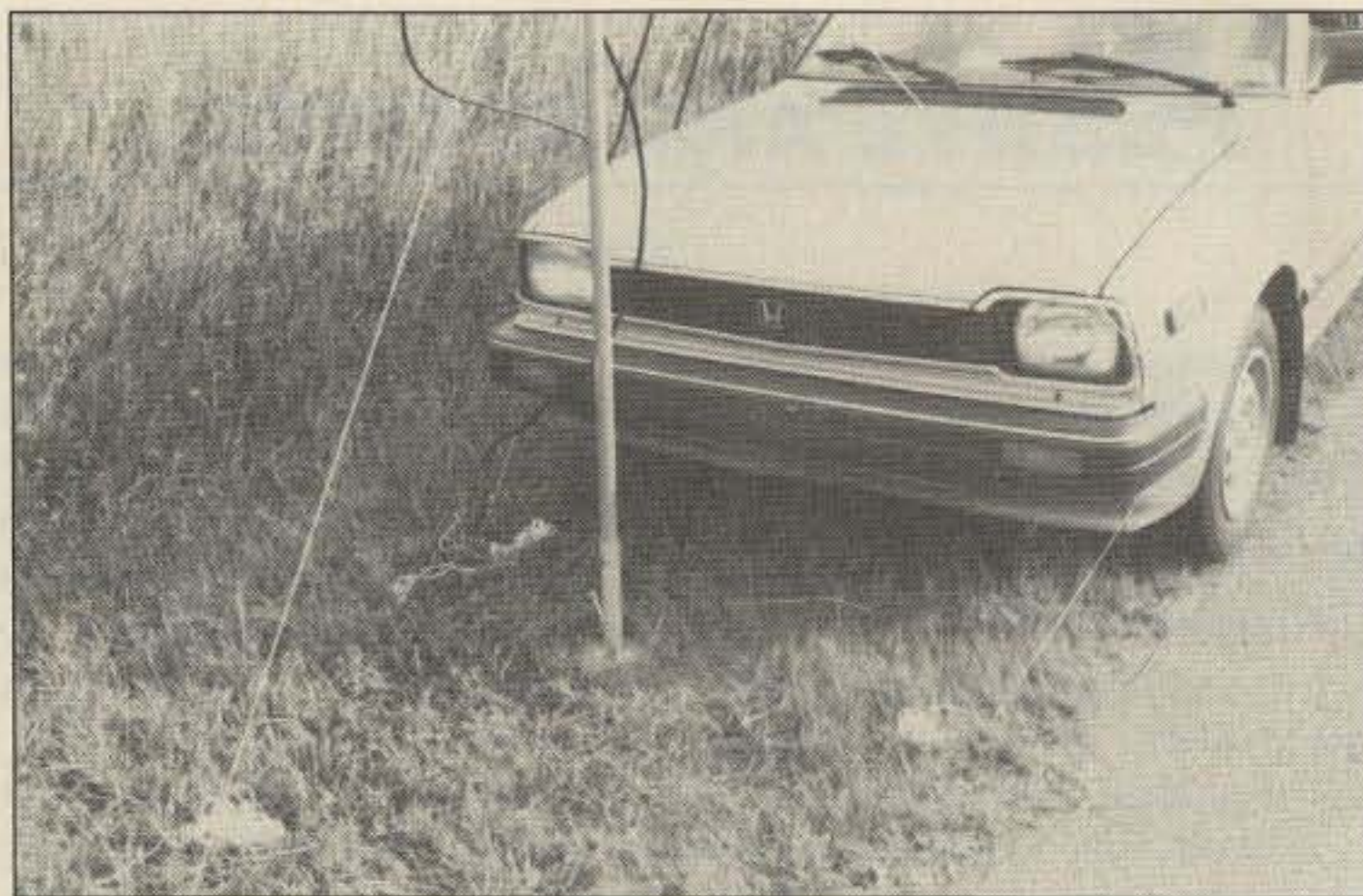
Photo C. Mast support plate and guy lines. The Honda makes a good anchor point!
