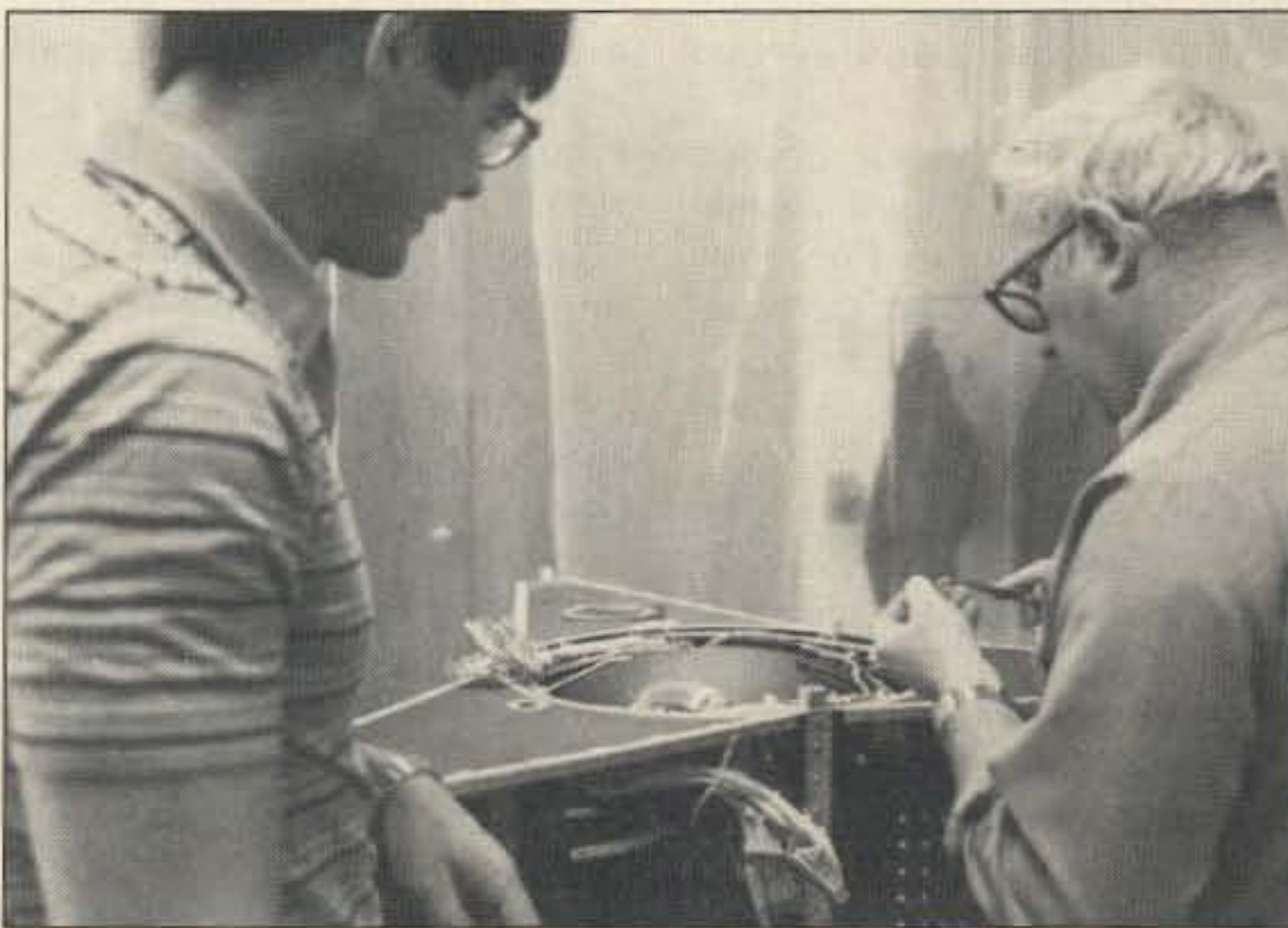
Photo A. OSCAR 13 spaceframe in construction in Colorado.
