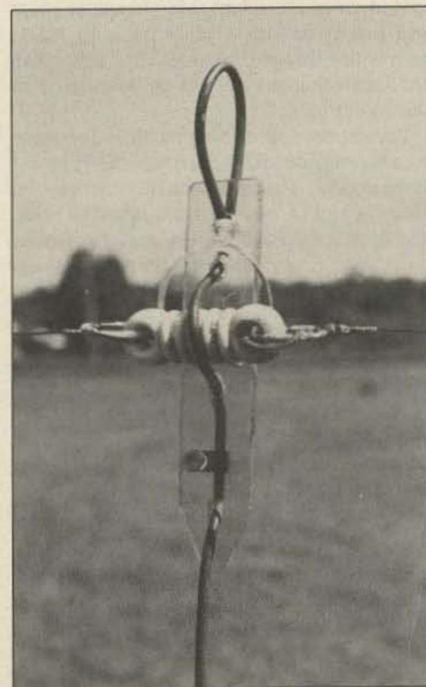
Photo D. Feedline protection using the PY8ZAC/W8VOH method.
