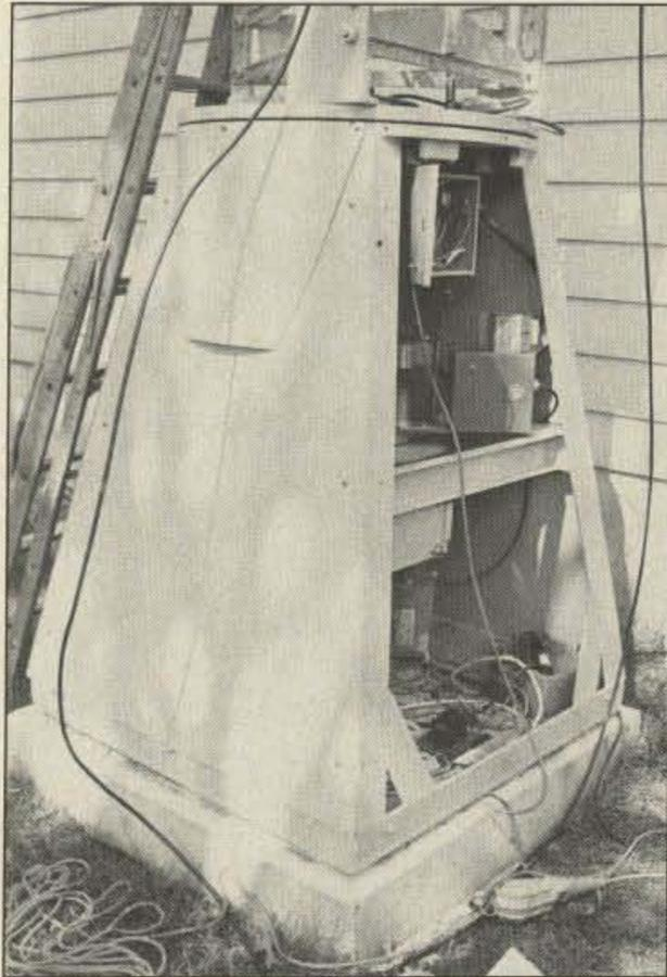
*Photo B. The base pedestal with the cover removed. The large concrete base is visible, as is the lazy-susan turntable at the top. (Photo by KT2B.)*
