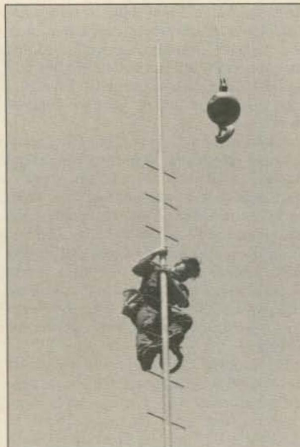
Photo E. The mast has just been installed with the help of a crane. WA2VUN is standing on Rebar steps. (Photo by WB2WIK.)
