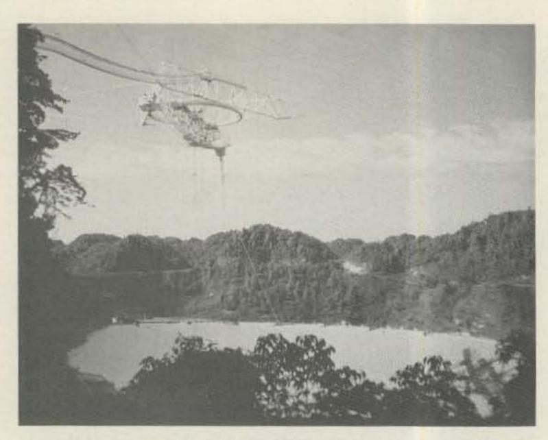
The platform structure weighs 600 tons. Most of the antennas which receive the signals that are reflected from the reflecting dish are mounted on two carriages which can move along the curved track on the underside of the platform.
