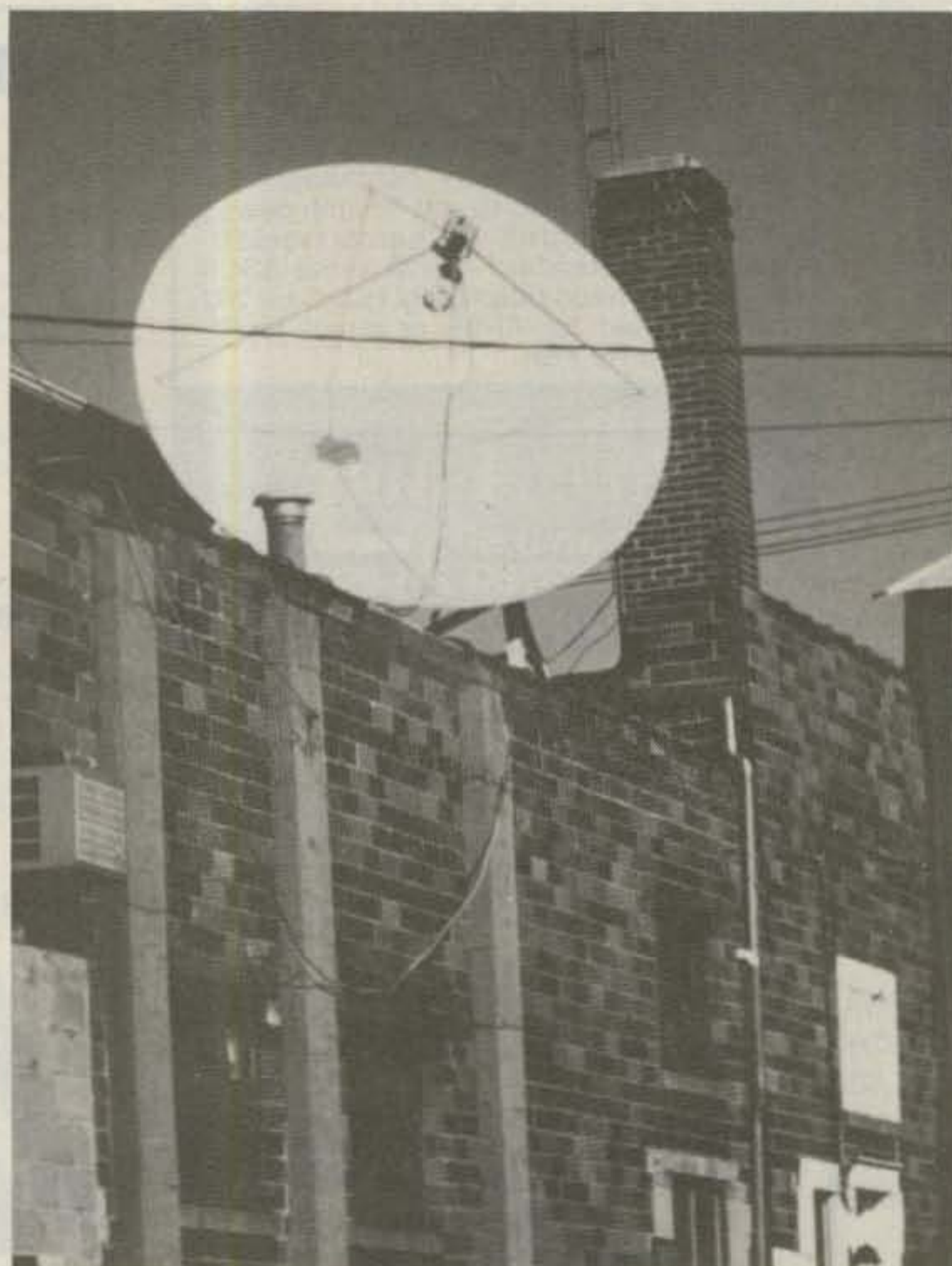
Photo C. If you can't find a suitable spot on the ground for your antenna, consider using a roof. It almost guarantees a clear shot at the satellites.
