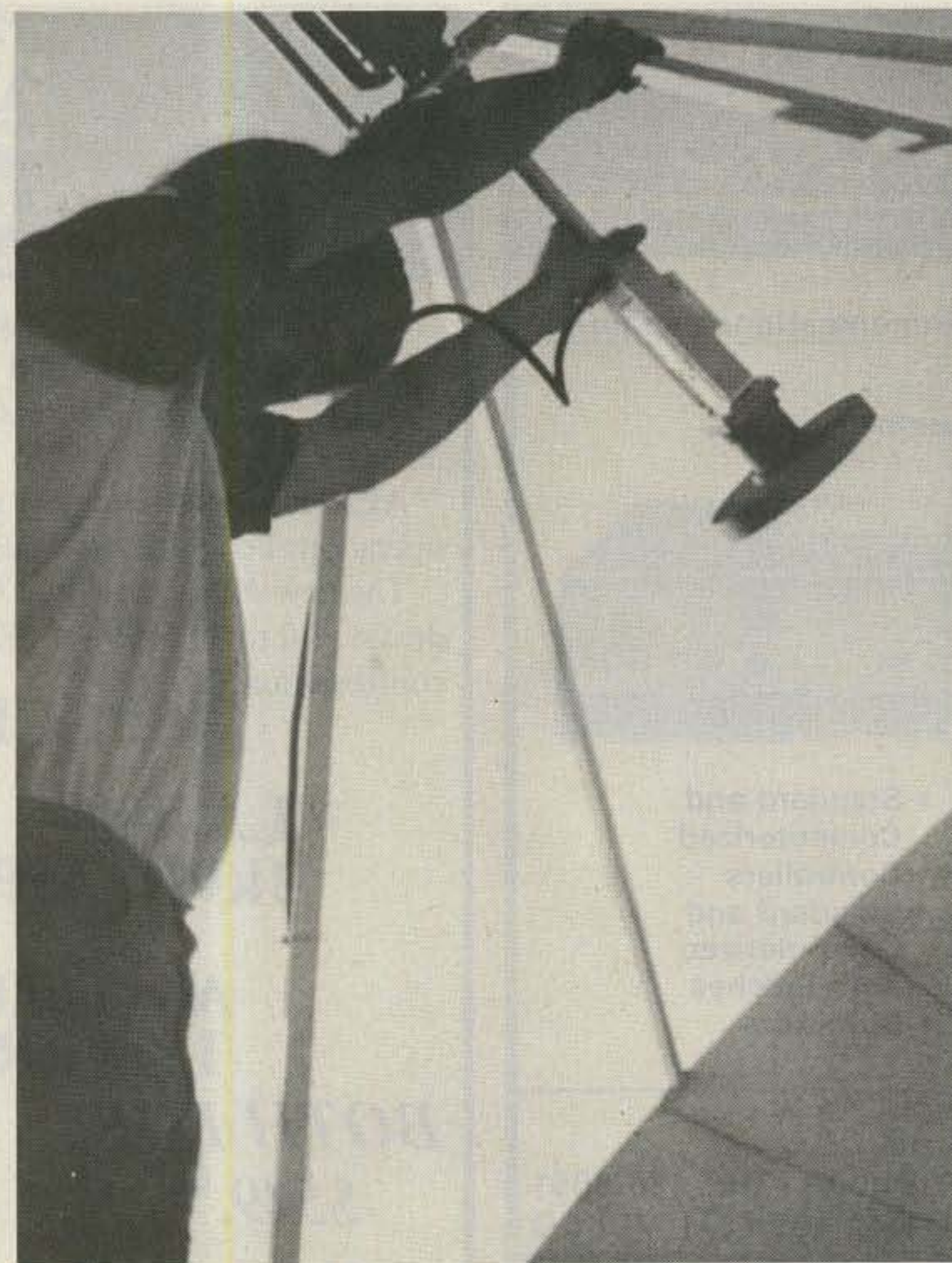
Photo D. Feedhorn placement is critical. Start by finding your antenna's focal point and then make slight variations in the feedhorn position until the signal is maximized.
