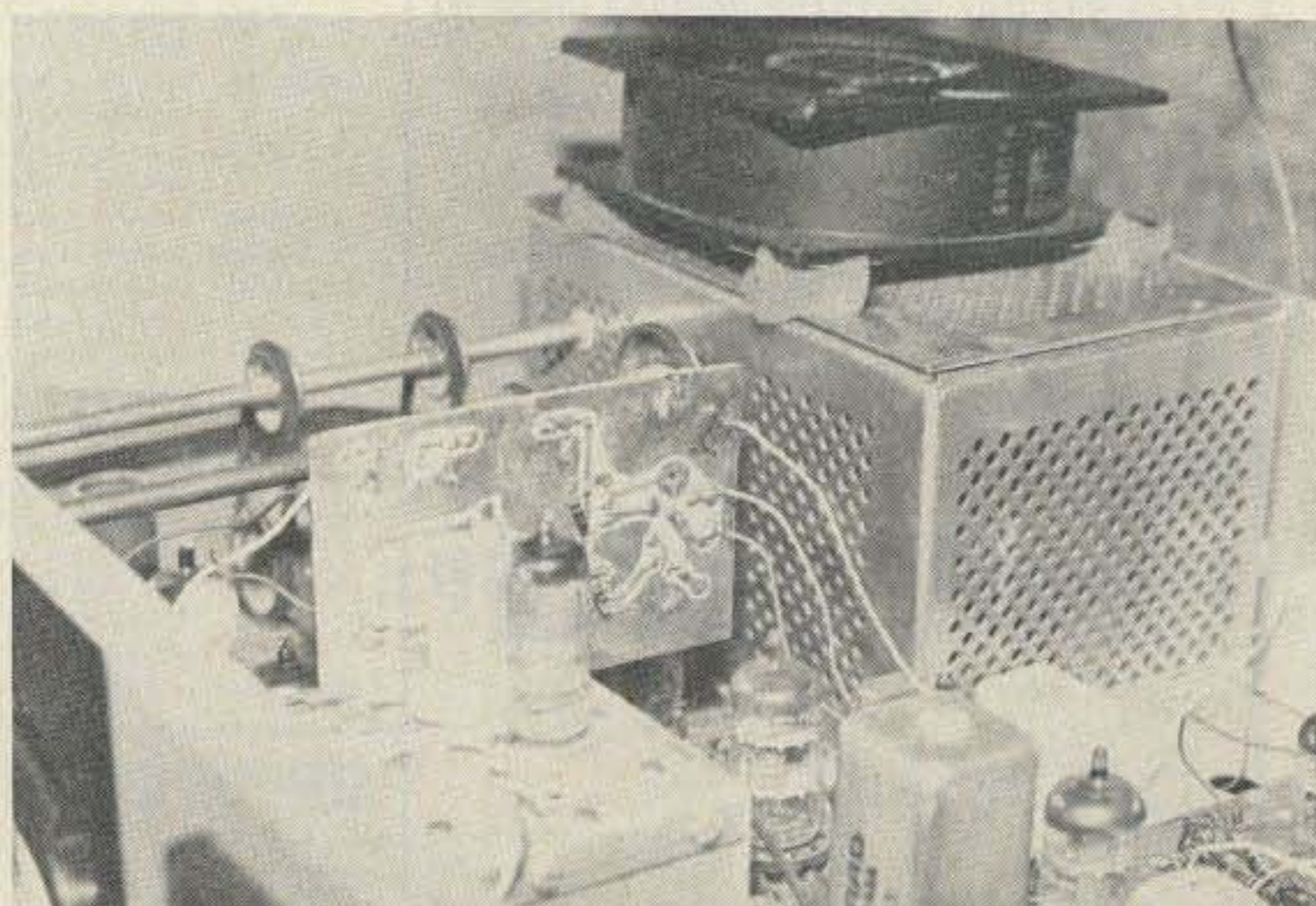
Photo B. Rear view of FSK board showing wires from computer.
