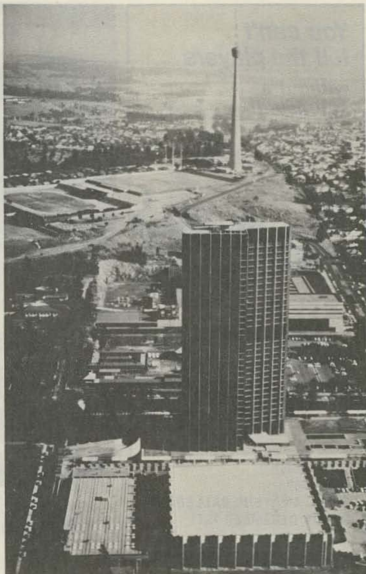
Broadcasting center of Radio RSA in Johannesburg. Large tower in back holds FM radio antenna.
