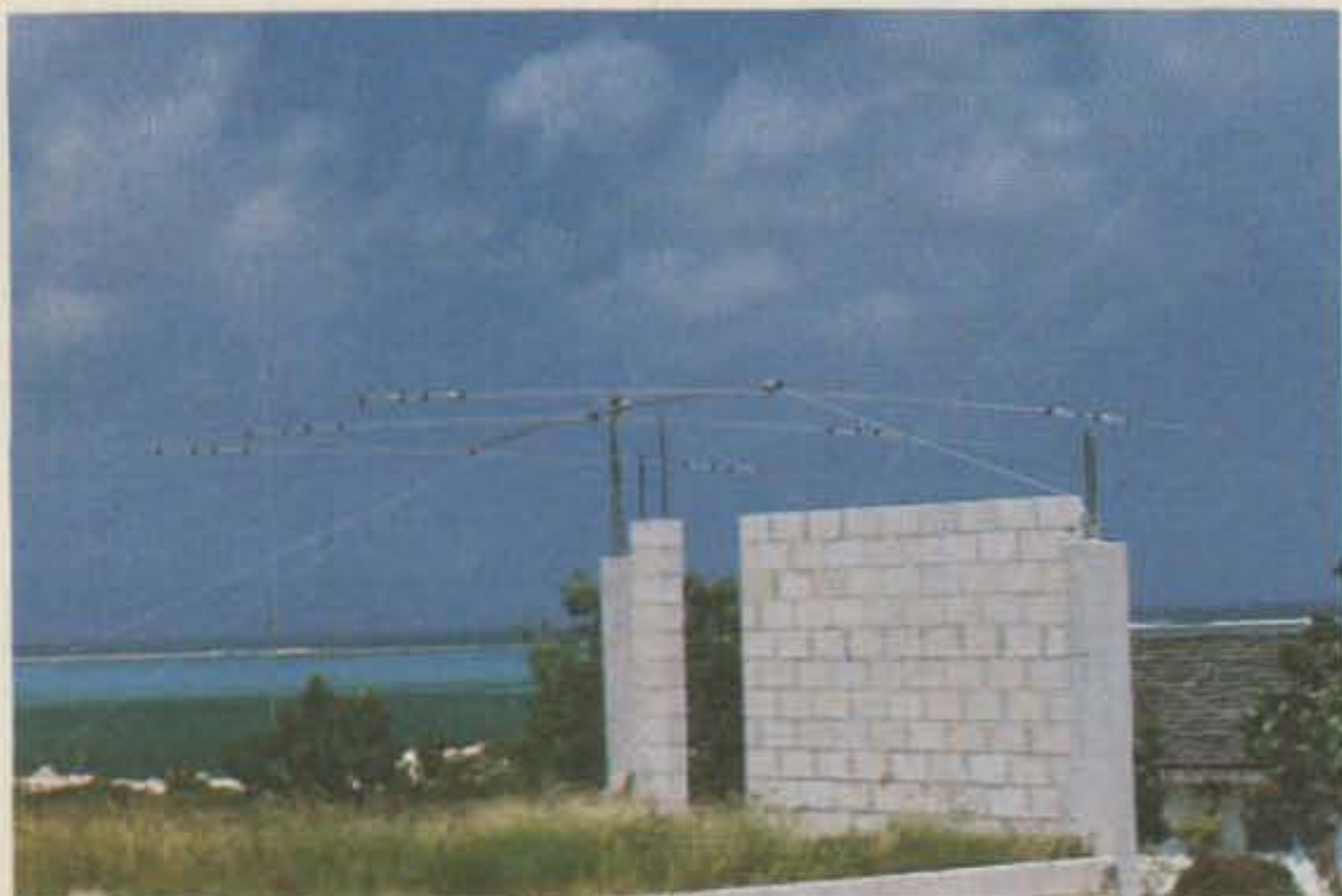
Once atop the wall, the antenna was tied off to prevent the ever-present tropical breezes from tearing it to pieces. Kansas is dead ahead.
