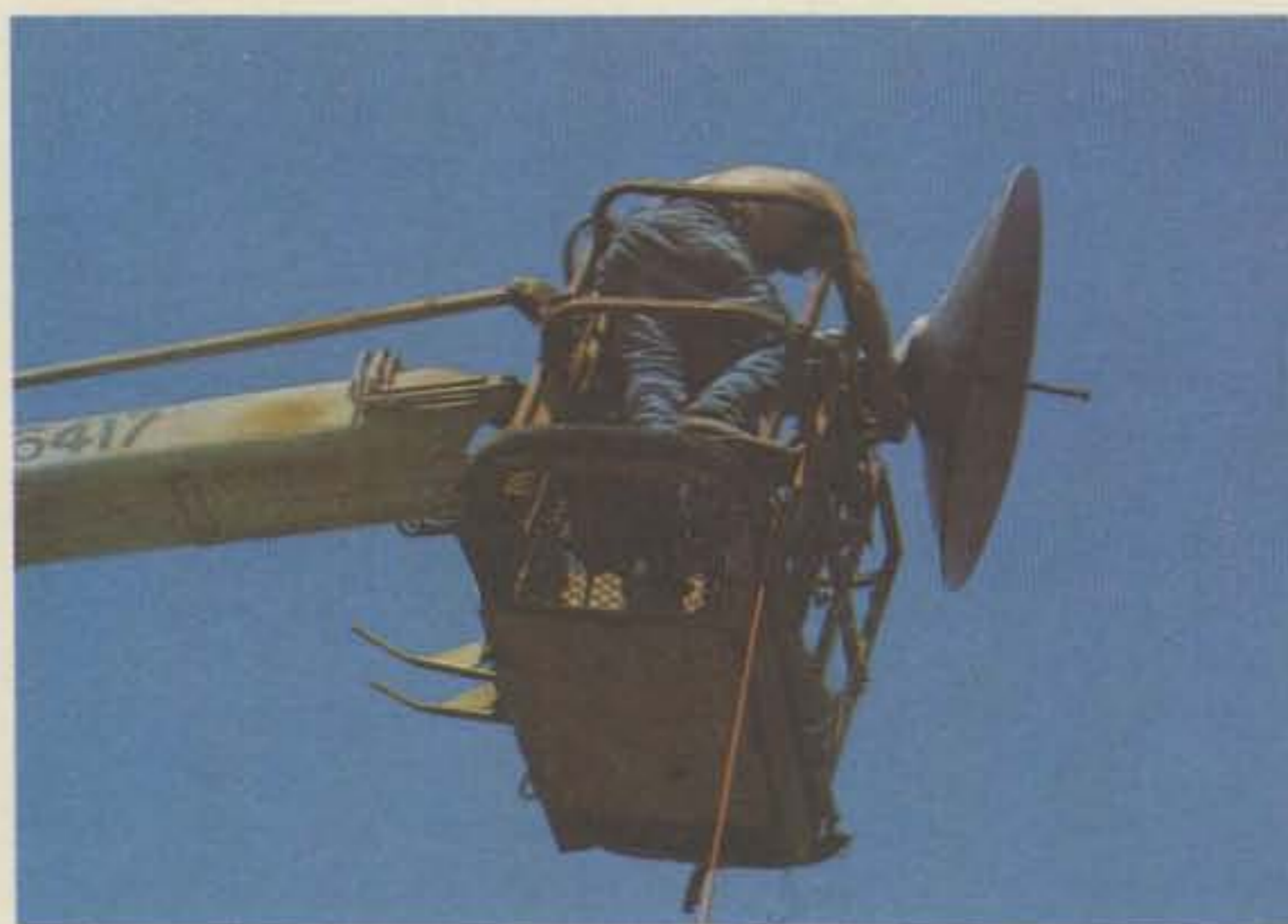
Up, up, and away. The cherry picker is pressed into service so that the microwave signals can clear the trees easily in all directions.
