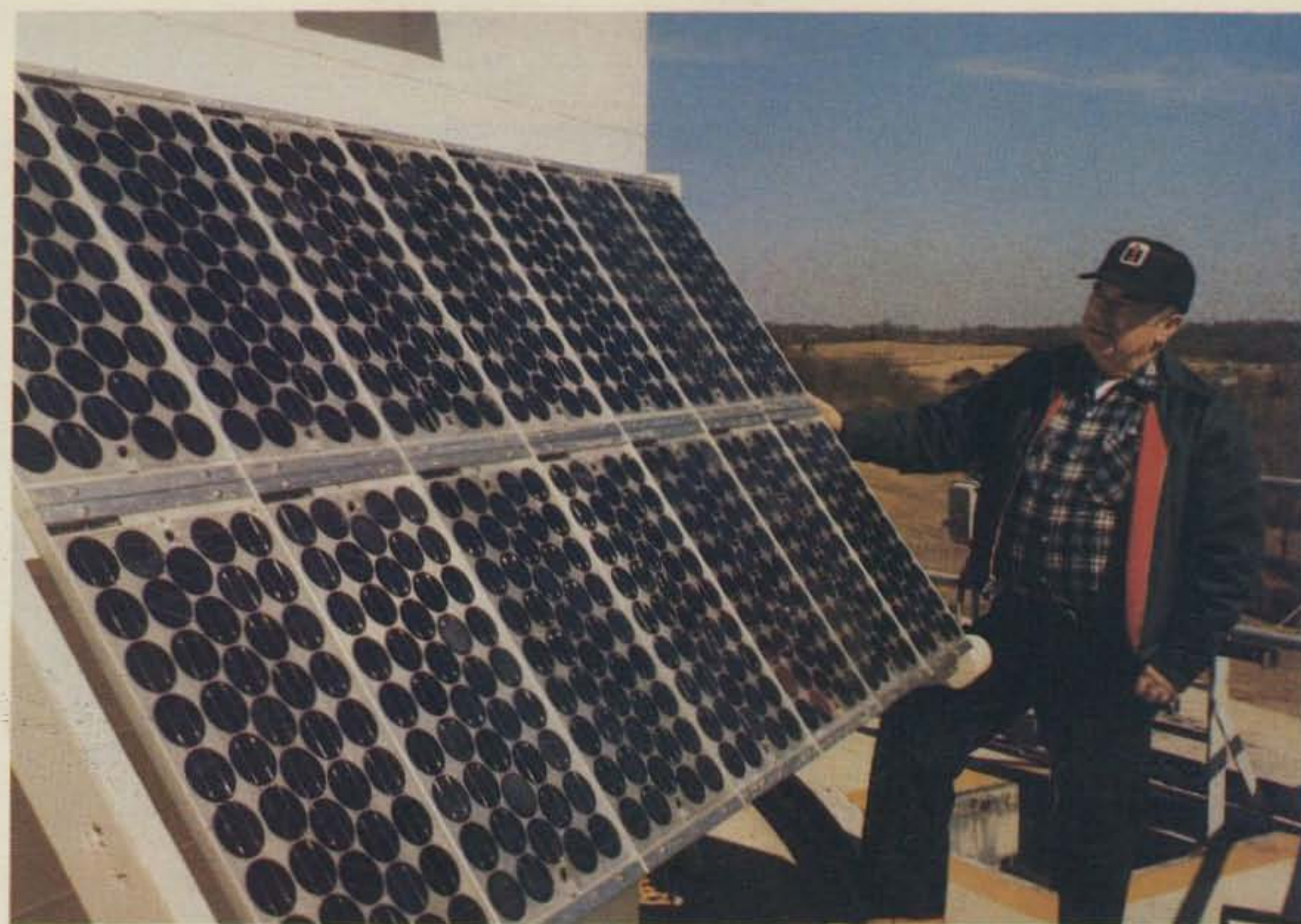
Photo B. Photovoltaic array. Frank Troutman WB3CLF helped install the array on the side of the shack.
