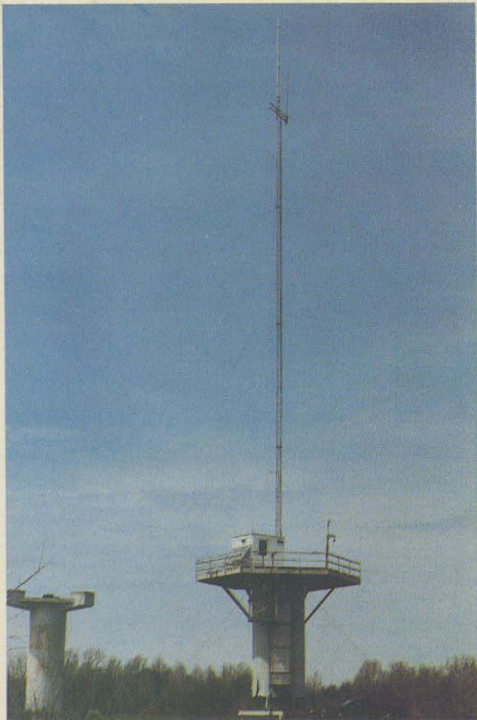
Photo A. AARC repeater. Photovoltaic array is visible on the left side of the shack at the base of the tower.
