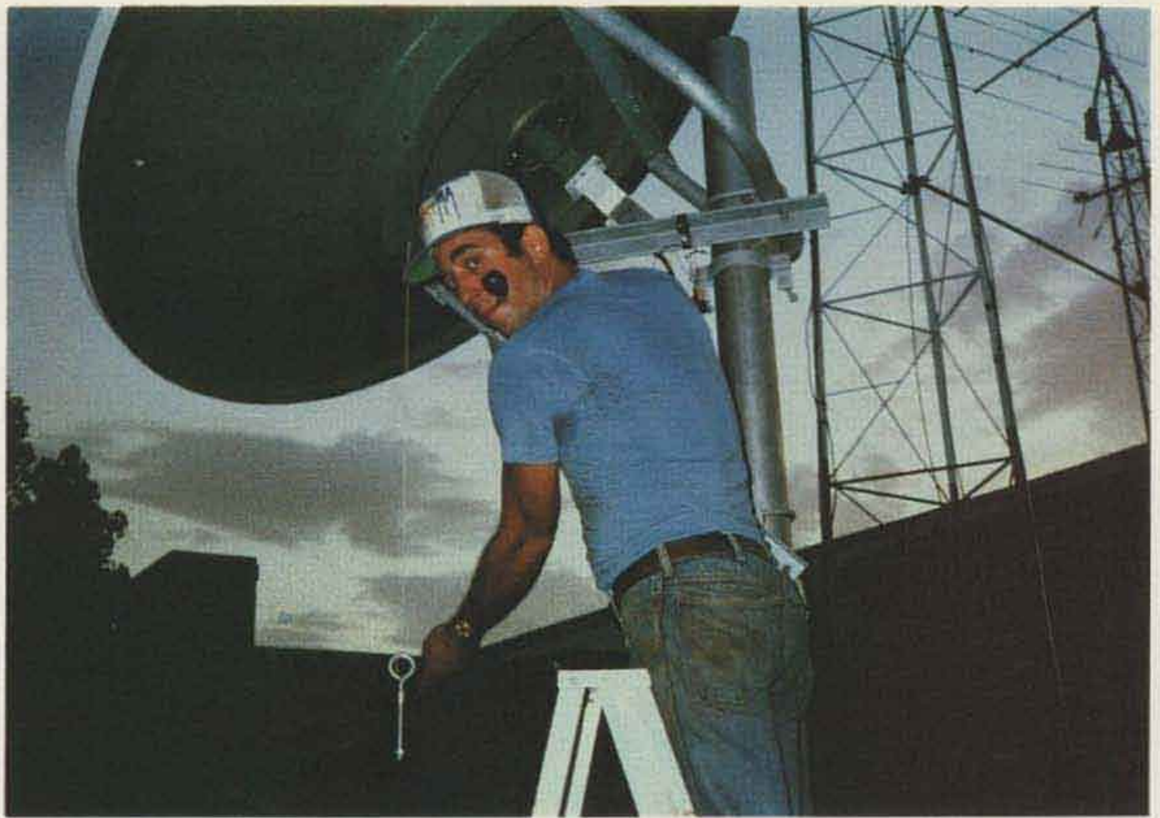
Photo H. The author checks the elevation angle on the six-foot satellite receive-terminal using a 29-cent protractor. The back of the dish presents a right angle to the feed, allowing use of a simple protractor with string and weight to check the elevation angle.
