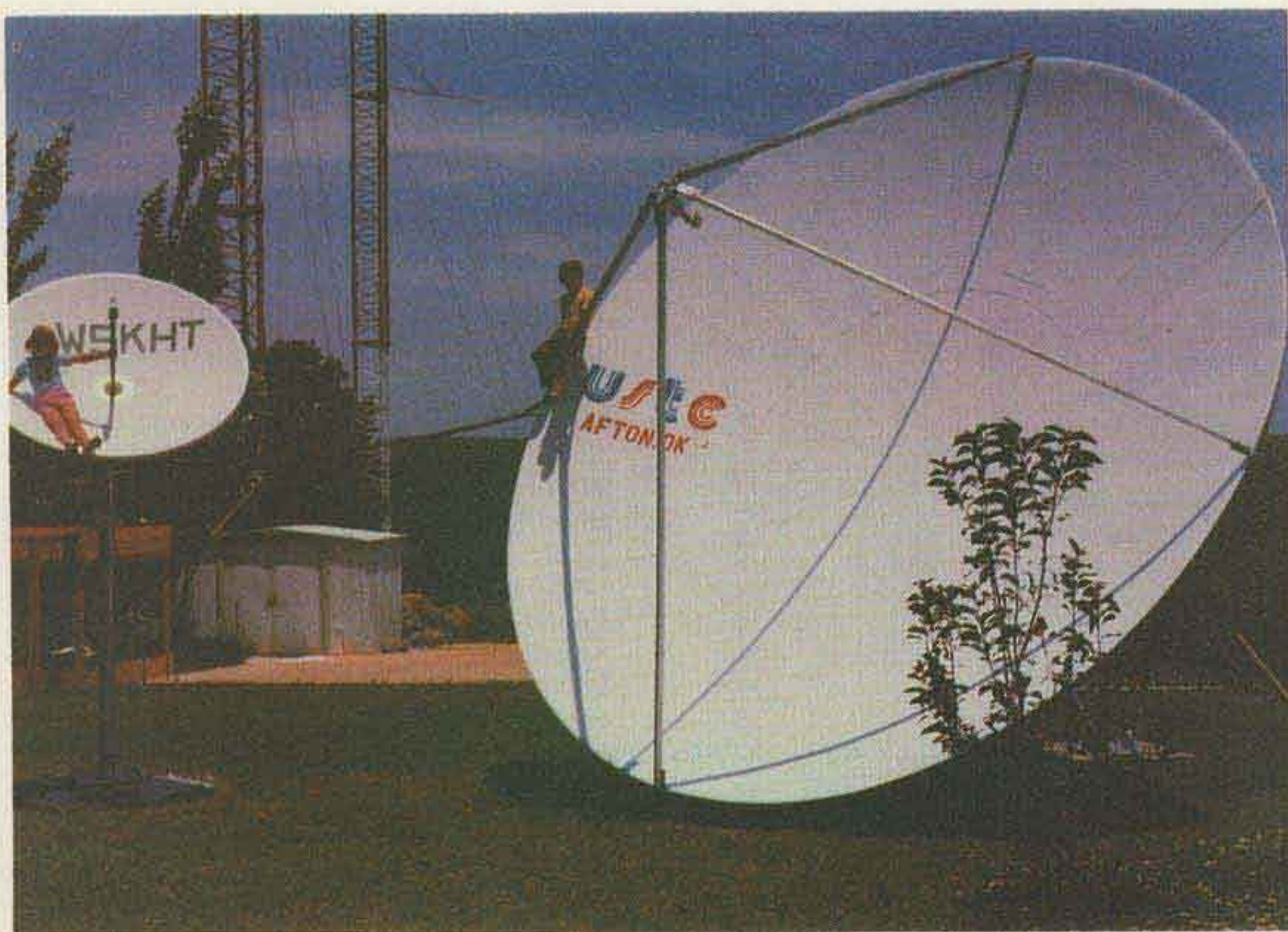
Photo G. Six-foot (left) and twenty-foot satellite antennas. The six-foot one is positioned on WESTAR I while the 20-foot one is on SATCOM F1. White reflective surface is essential to keep the sun's rays from "cooking" feed (and electronics there).
