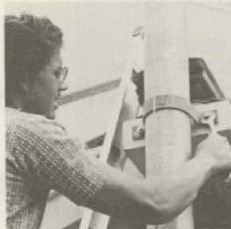
Mounting the House Bracket
