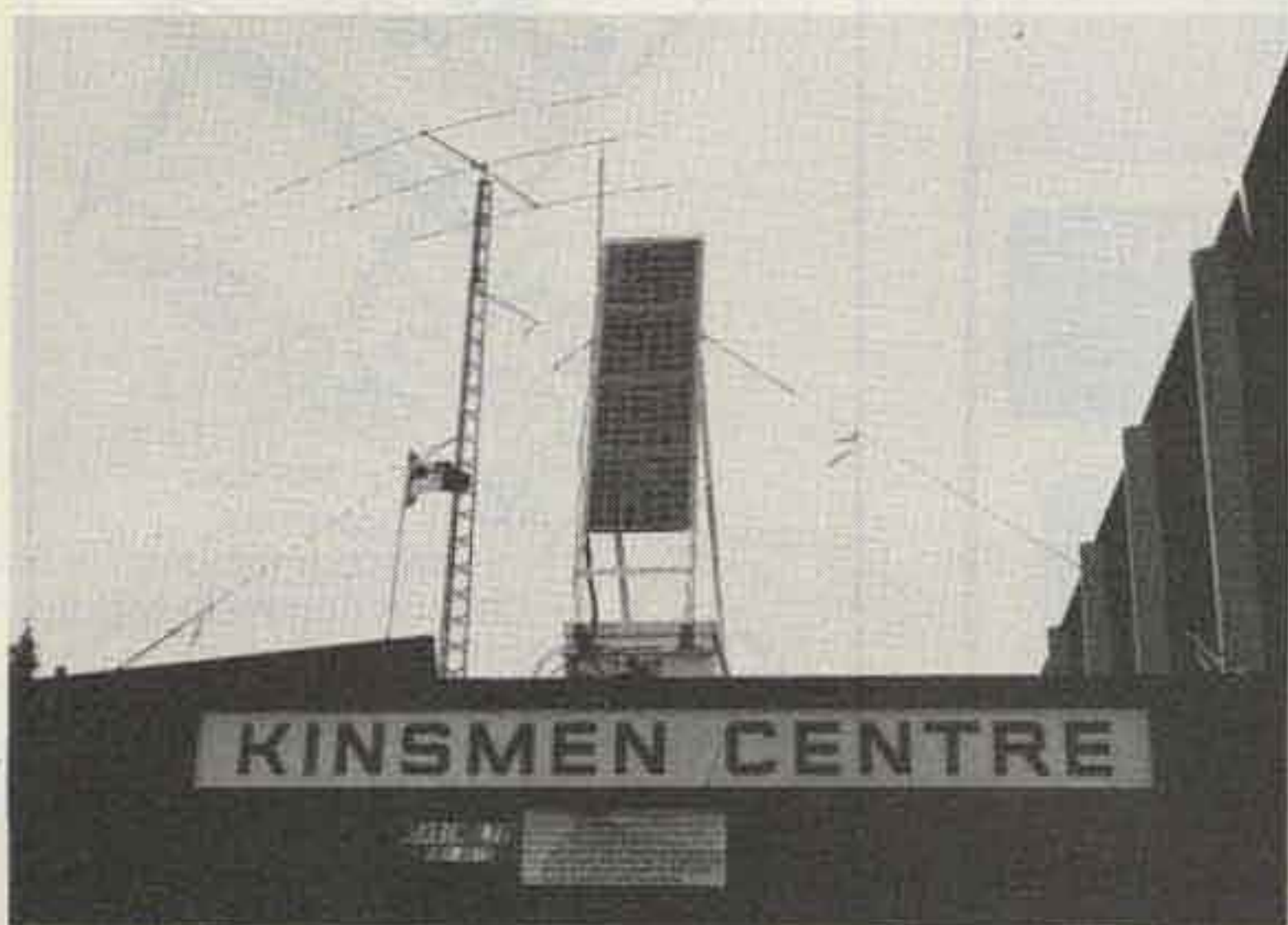
The power supply and tribander up on the roof of the exhibition building housing the station. The solar panels shown provided enough power to keep the six 105-Amp batteries stored at the base of the panels always close to full charge.
