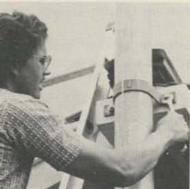
Mounting the House Bracket
