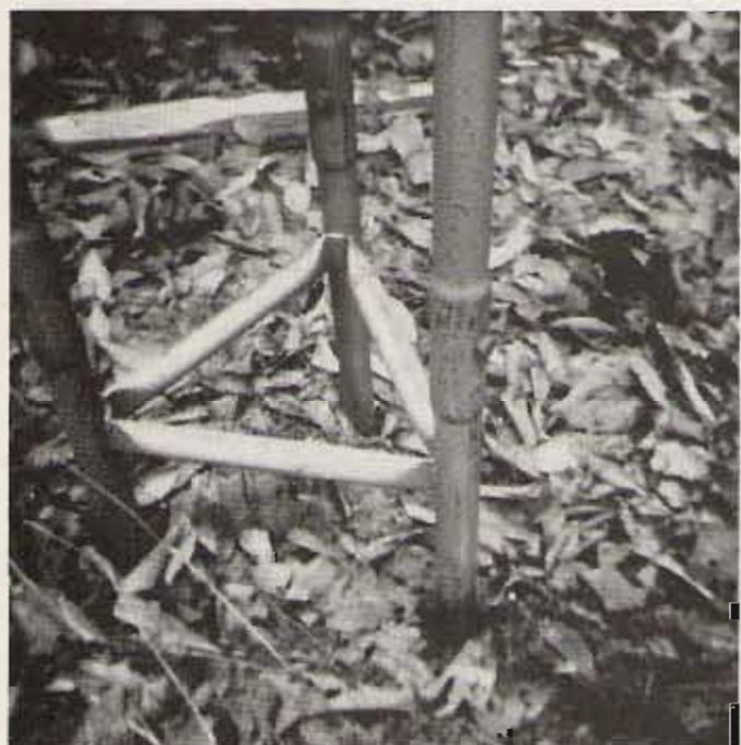
The Dill tower base rests on a large flat rock two feet down and buried in small rocks and well-tamped dirt.
