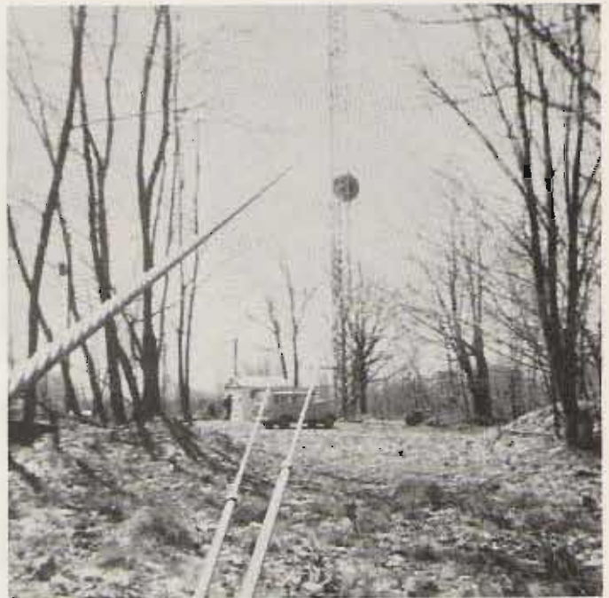
The bottom two guys shown here are attached to the anchor plate and to the "star mount" just below the microwave dish.
