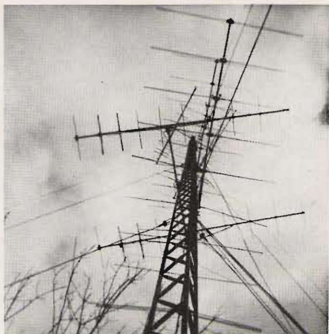
A Dill tower in CATV service is pictured here. The tower is 100 feet tall, in 10 foot sections weighing about 60 pounds each. The sections are 11 inches on a side.
