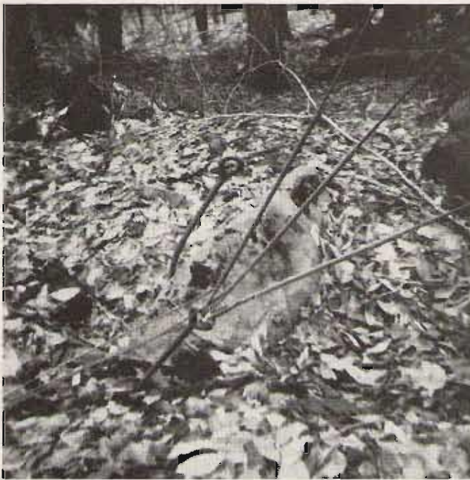
The anchor rod holds three guys using preformed grips. The rod is six feet long and is buried nearly five feet down.
