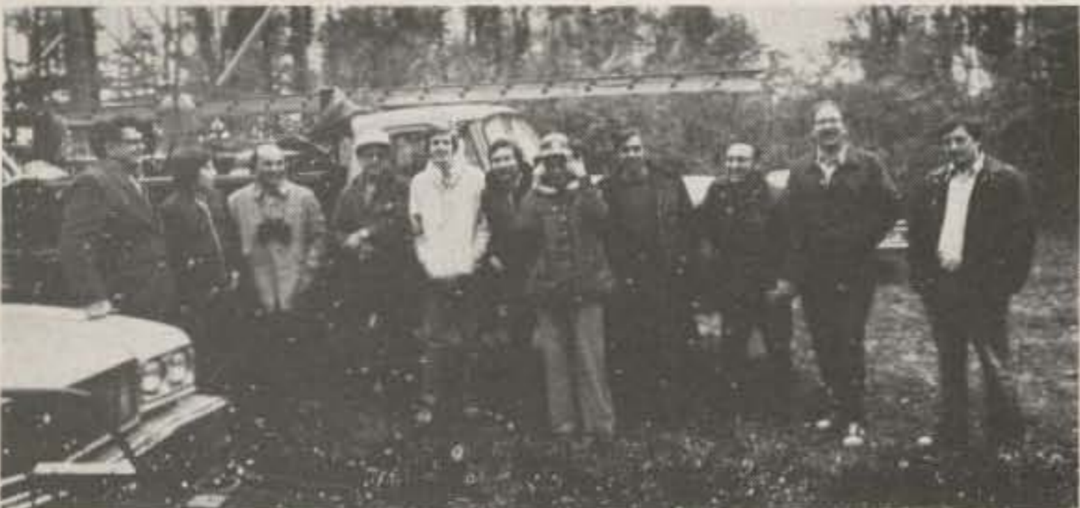
Last November, LIMARC (Long Island Mobile Amateur Radio Club) members erected three new ATV repeater antennas at their new Syosset, New York, site. The installation crew included (left to right) WB2KCD, WN2VVR, W2MVS, W2KPQ, KA2CLQ, W2TRP, WA2SHC, WB2WAK, N2FP, K2LIO, and WB2SDG. (Photo by K2JKX)
