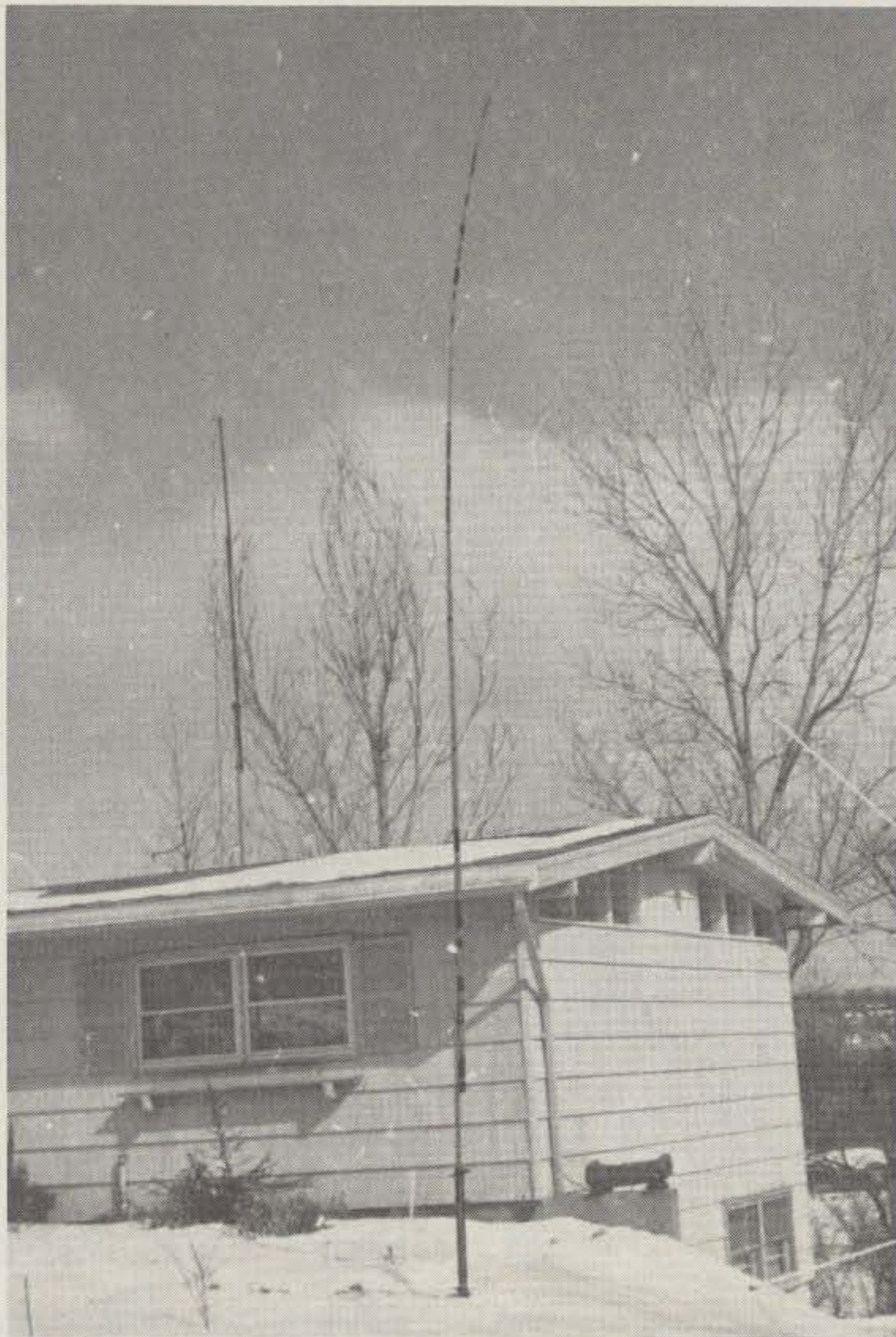
"Vertical zepp" antenna for 20 meter CW.
