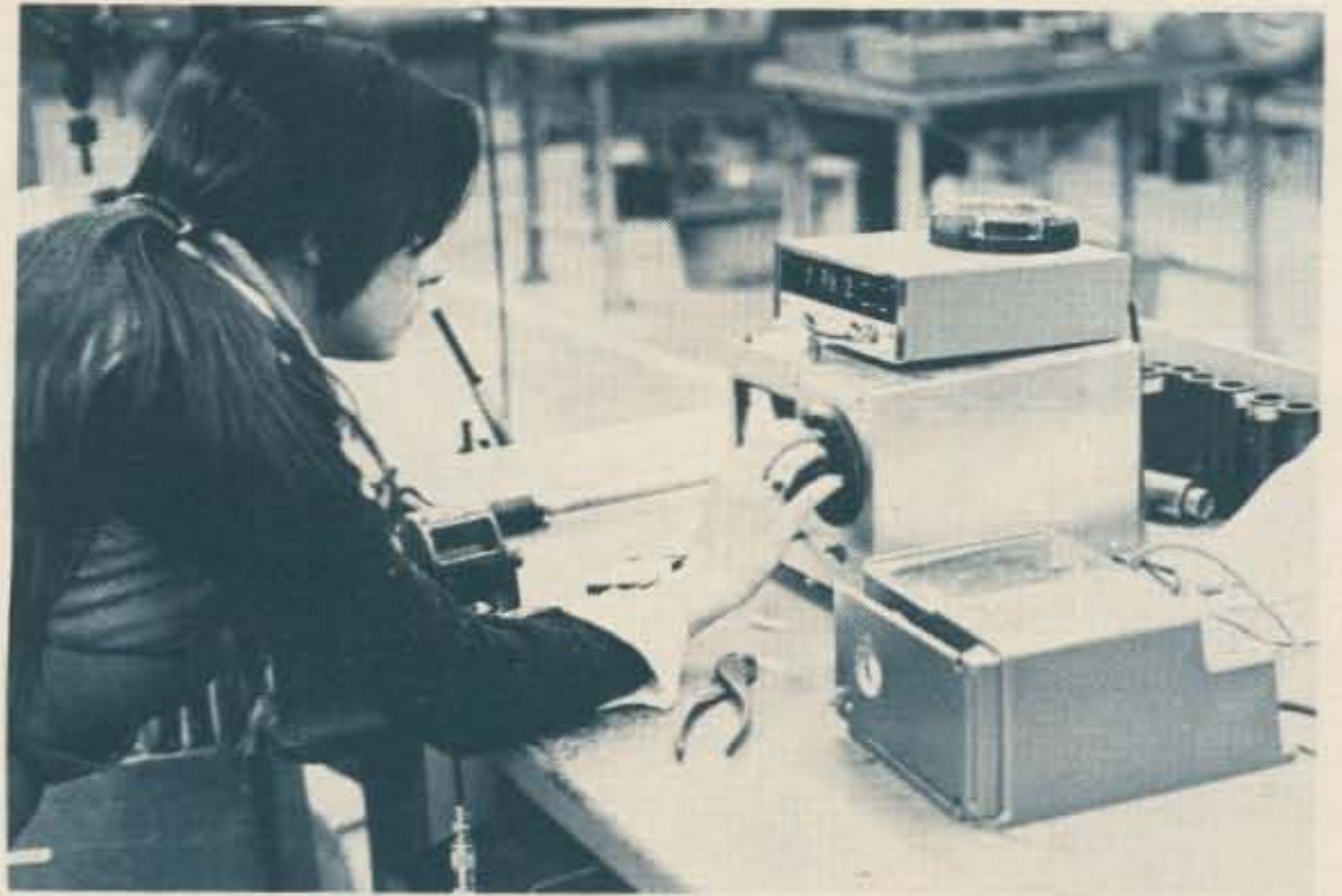
Debbie Narcos is checking the pruning of a coil with an oscillator and frequency counter. They come to her a bit low in frequency, and she gets them right on with the coaxial cable "pencil sharpener" next to her hand.
