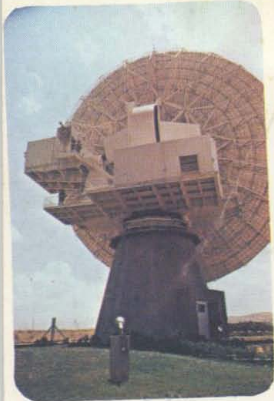
Telephone and TV via Satellite
