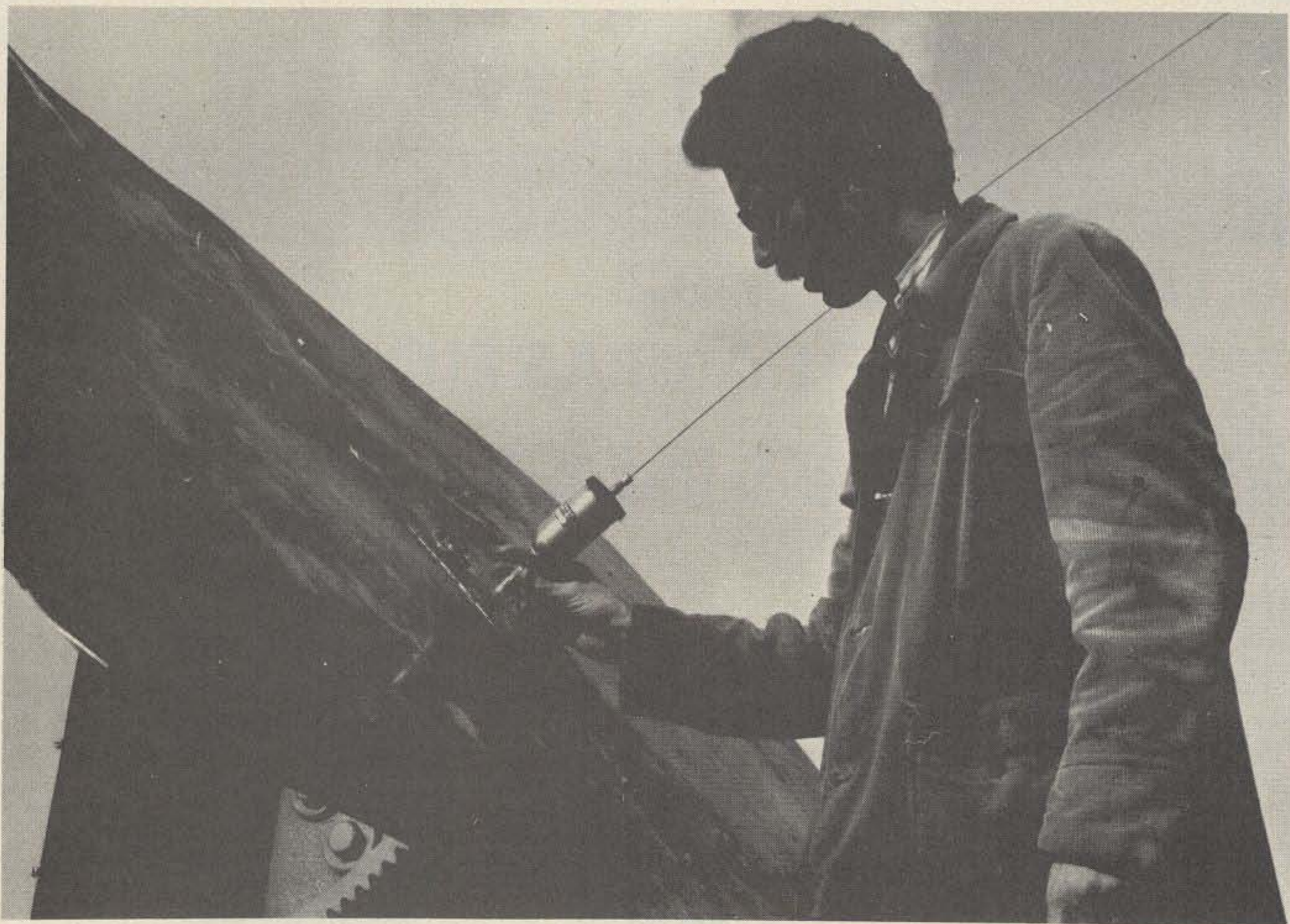
\frac{1}{2}\lambda Gam mounted-on ground plane.
